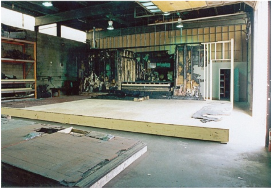
West end of club, reconstructed in evidence warehouse. Note downward-sloping tile floor in foreground, recovered from front entrance to The Station. (Photos, William White)
