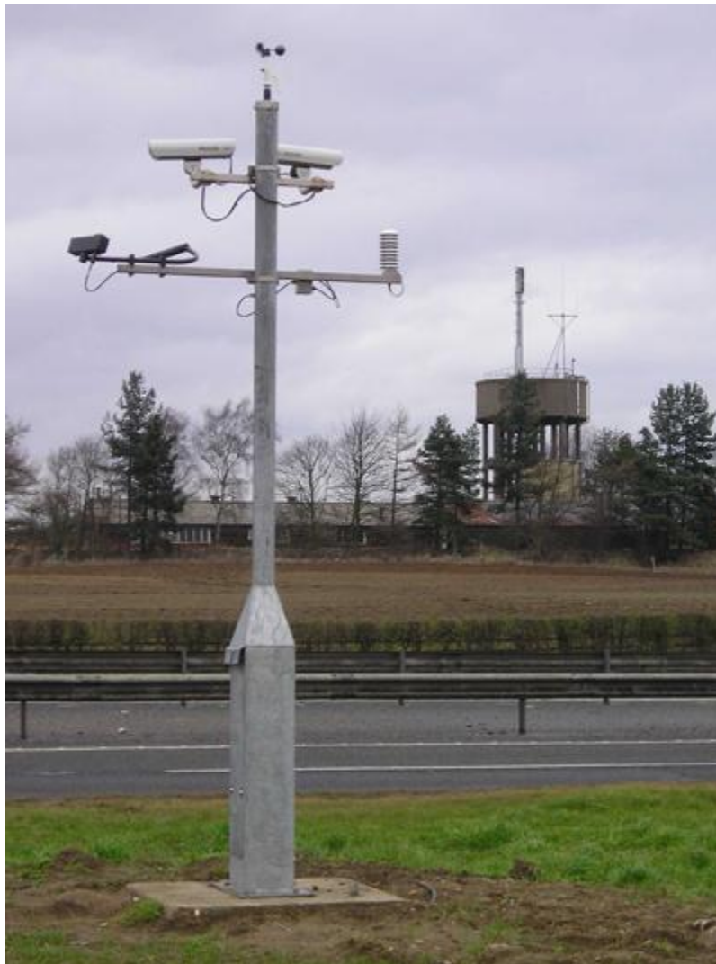
Figure 3.4. This weather station transmits data about the weather and road surface conditions to IceBreaker, which uses the information to predict ice formation. These predictions are used to dispatch trucks to treat the roads with de-icing material. Photo of Vaisala Weather Station ROSA courtesy of Vaisala. www.vaisala.com ( http://www.vaisala.com ).
