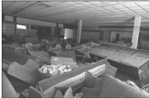
FIGURE 2-4: Mullens, WV, July 17, 2001. An office supply store is in shambles after floodwaters up to 9 feet hit earlier this month. (Photo by Leif Skoogfors/FEMA News Photo.)
